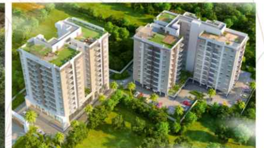
GOLDEN WOODS UMANG Jyoti Nagar, Panigaon, Nagaon
